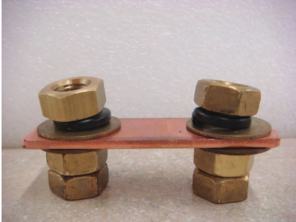
Photo shows extra nuts installed under jumper bar for clearance of power bolt Insulation
