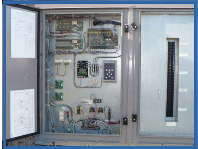
Panel mounted MCS Controls on Carrier Chiller
