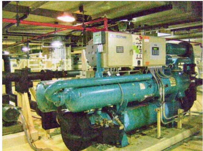
TVA Chiller with MCS Controls
