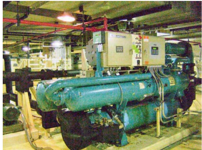
TVA Chiller with MCS Controls
