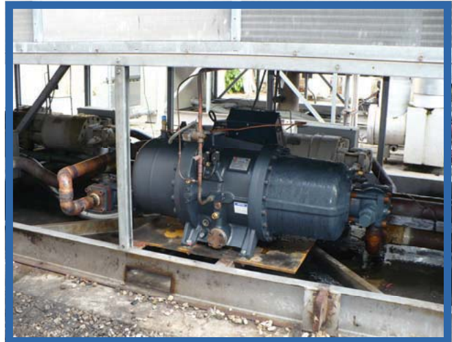
Hanbell RC15LF Compressor replacing Trane screw compressor on a Trane RTAA Chiller
