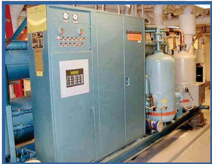
Dunham-Bush Chiller with MCS Controls in a door mount application at G.E. Corporate Head Quarters.
